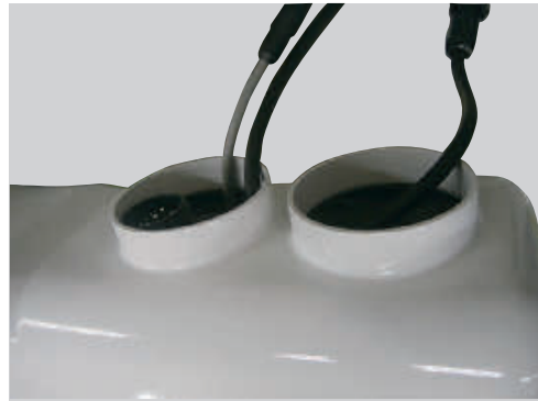
Cables removed when temporarily inserting cover
